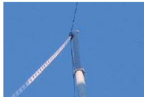
At the top of the feeder, after weather-proofing - not pretty but waterproof!!
