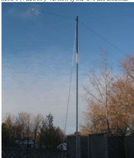
A good tidy G7FEK installation . This neat and tidy job is by Scott, VE3SCP. This is a 24ft vertical section with 8 and 38ft horizontal extensions.
