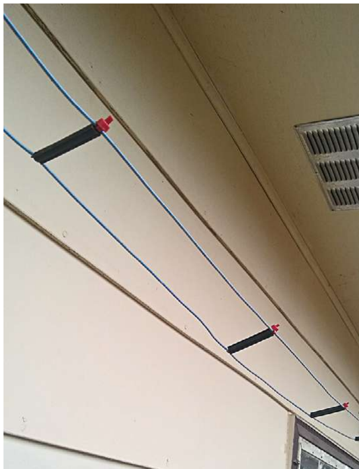
The doublet’s “integral” ladder line feeder is made from THHN house wire, tubular electric fence insulators, and UV-stabilized zip ties. This design is rugged, weathers perfectly, and works flawlessly. I will use it again as necessary. (NT0Z photo)
