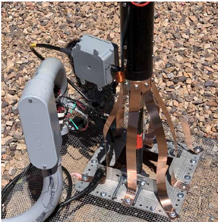
Scorpion installation of Steve Reed KW4H showing square balun, copper grounding straps, and DX Engineering radial plate. Wire mesh acts as the radial ground field. The small copper coil in the center is called a shunt coil (between hot and ground side of antenna). Ideally, the wire mesh radial field should equal the height of the antenna (about 12 feet with the Scorpion). (KW4H photo)
