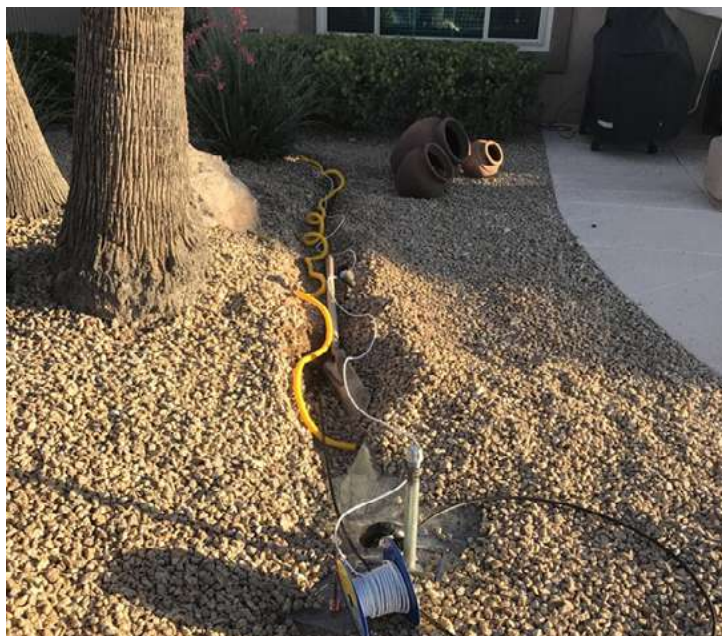
The author used yellow split-loom tubing to protect the coax and signal cables in our Arizona rock lawns. The trench is about 4-5" deep. Others have run 1-1/2-inch or 2-inch PVC conduits for the cable run to the shack. The wire mesh radial field has already been covered up in this photo. Note the steel water pipe where the Scorpion will be mounted. (NW7D photo)
